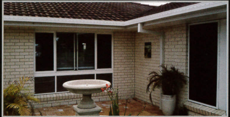
After - Home fitted with Xceed perforated aluminium screens
